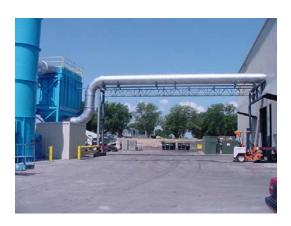
The RTO processes 25,000 actual cubic feet per minute (ACFM) of air containing approximately 250 parts per million (ppm) of CO and destroys over 95% of the CO produced by the new production lines. The system has been operational since May 2002 and has passed compliance verification testing.
